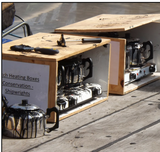
Hot pitch for the re-caulking
